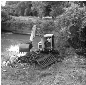
Works being made to clear the debris from the River Lark and removed the decommissioned bridge.
